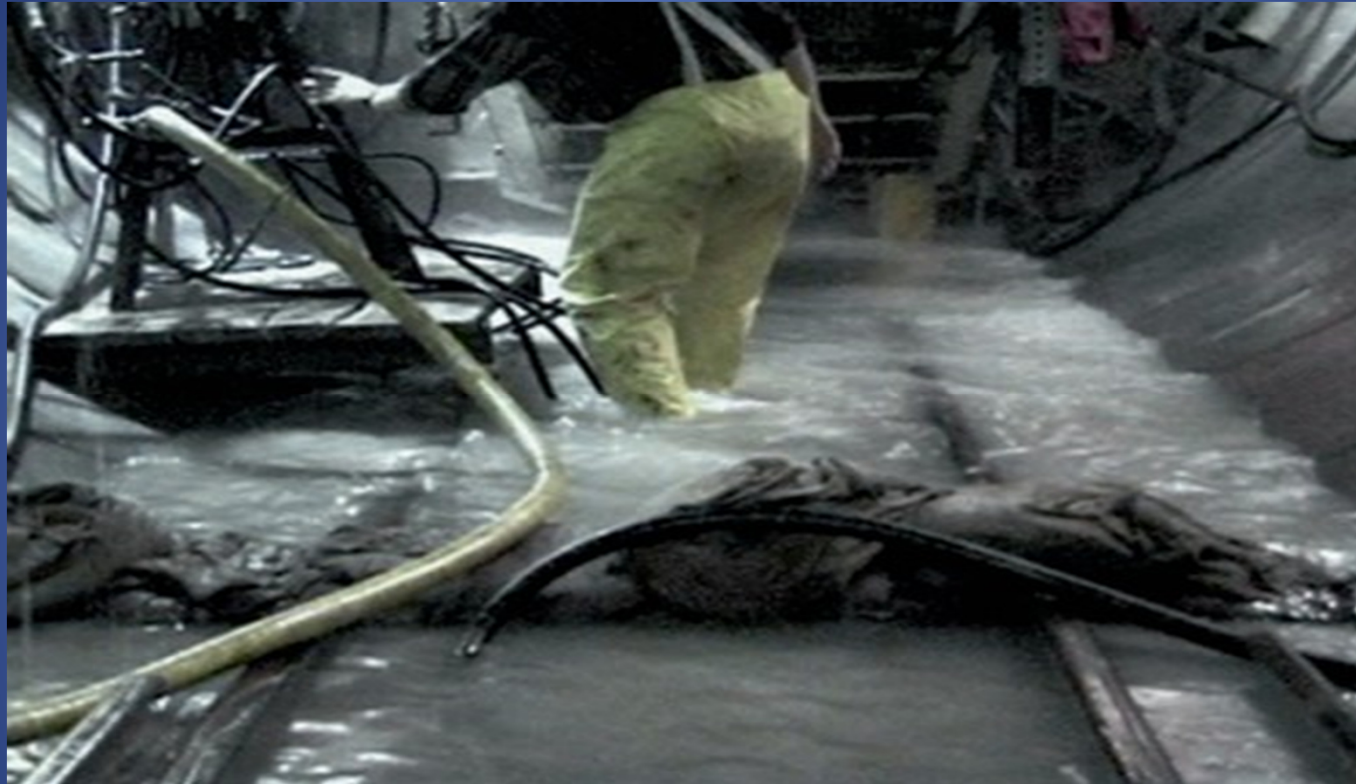
Groundwater inflows during tunneling
