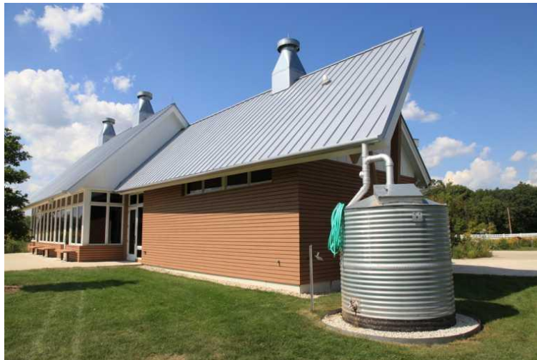
Figure 1. Picture of a rainwater rooftop collection system with an outdoor, aboveground storage tank. Notice that the gutter drainage includes a first flush diverter (the portion of pipe bypassing the storage tank). 1
